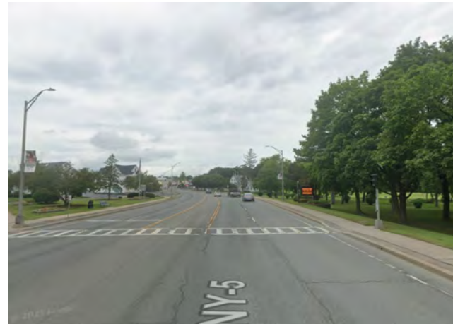
Existing Conditions on Mohawk Ave
